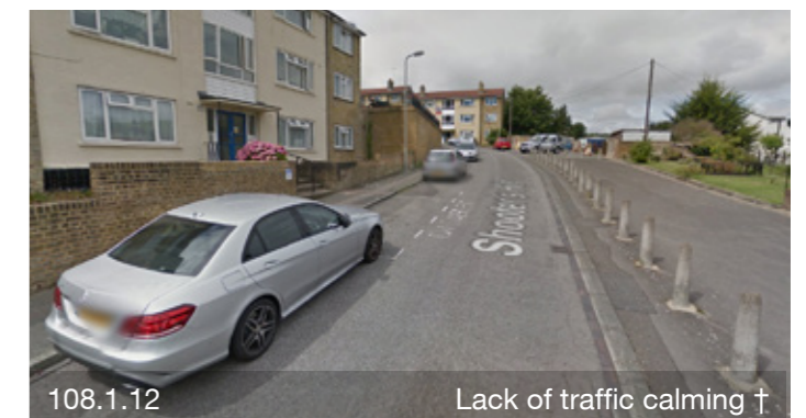
108.1.11 Poor transition from path to road
