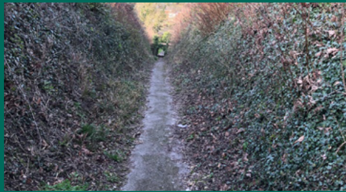
107.1.9 Poor surface condition
