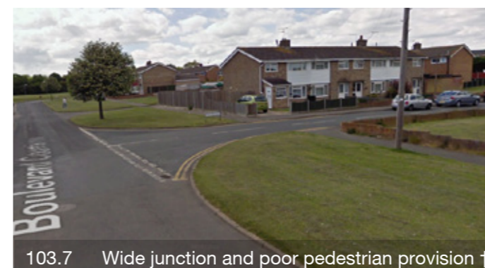
103.6 Lack of contraflow facility for northbound cycles
