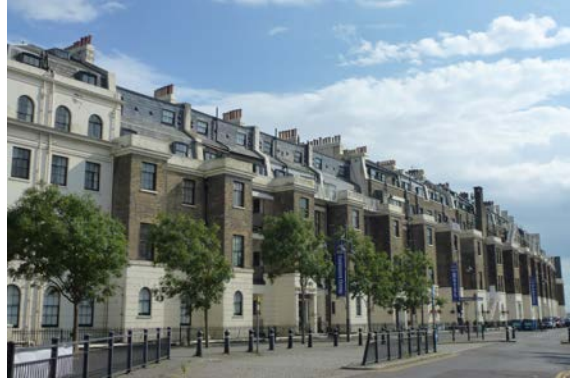
Waterloo Mansions - rear elevation
