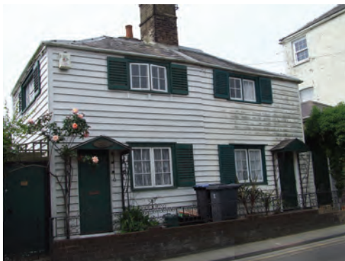
One of the few weatherboarded buildings in the conservation area.
