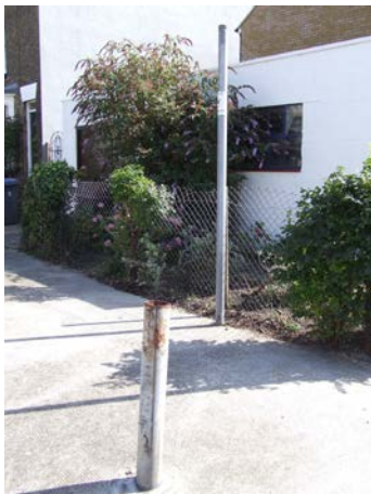
Redundant bollard and signpost
