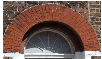
Typical features above a doorway
