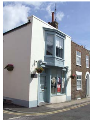
One of the few commercial premises (Duke Street)
