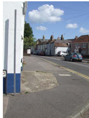
Pavement tarmacked in West Street
